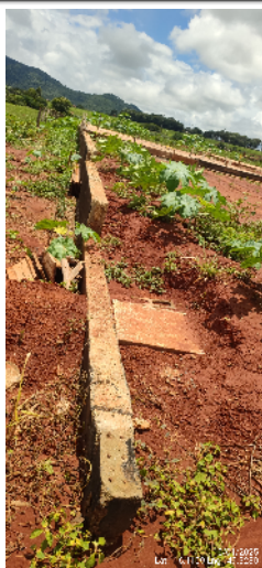
94-Muro de arrimo - LT 6 - Qd 16 10/01/25 12:28:18
